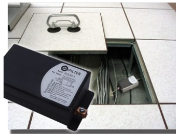
Facility ground under raised floor
